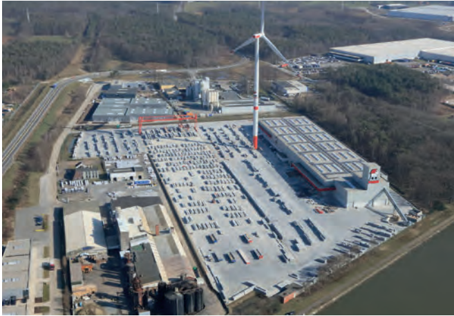
Aerial view of the Fingo production site in Tessenderlo
