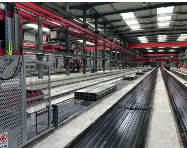
Stacks of hollow core slabs made by the stacker machine along the casting bed
