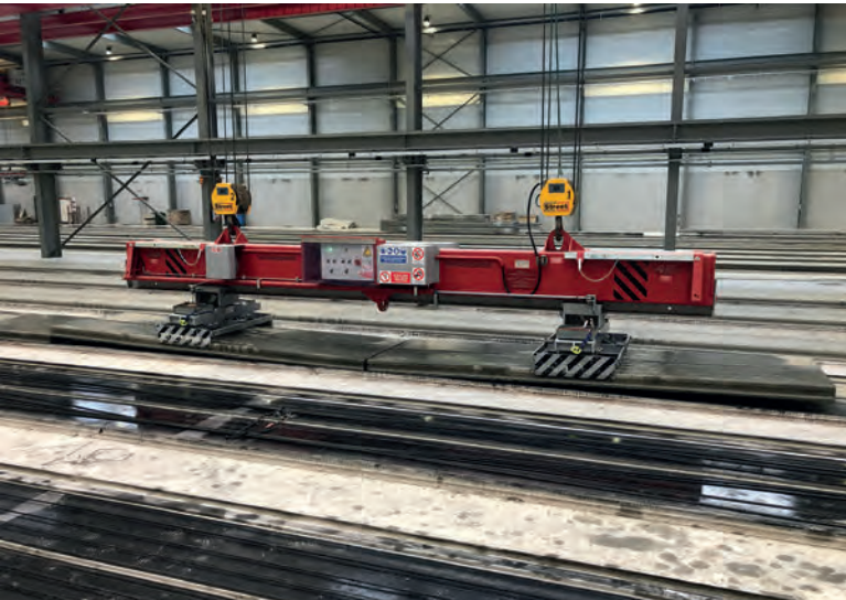
Hollow core slabs being lifted by a telescopic lifting beam and overhead crane
